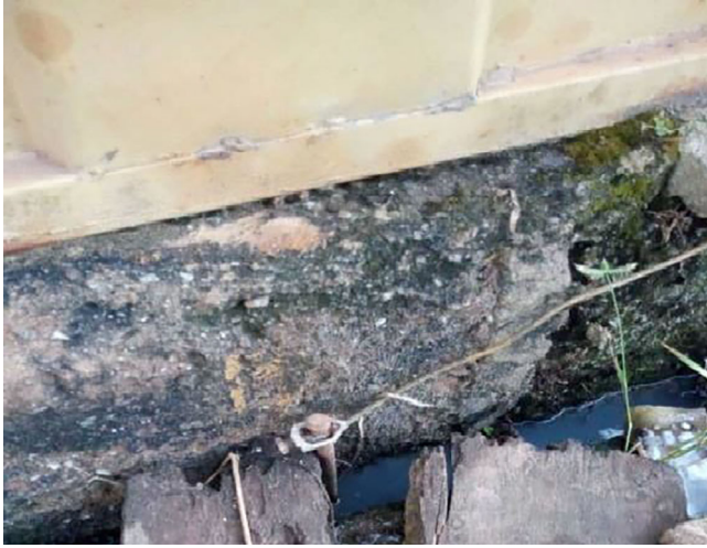
FIGURE 7 An electrode buried in a water log environment
